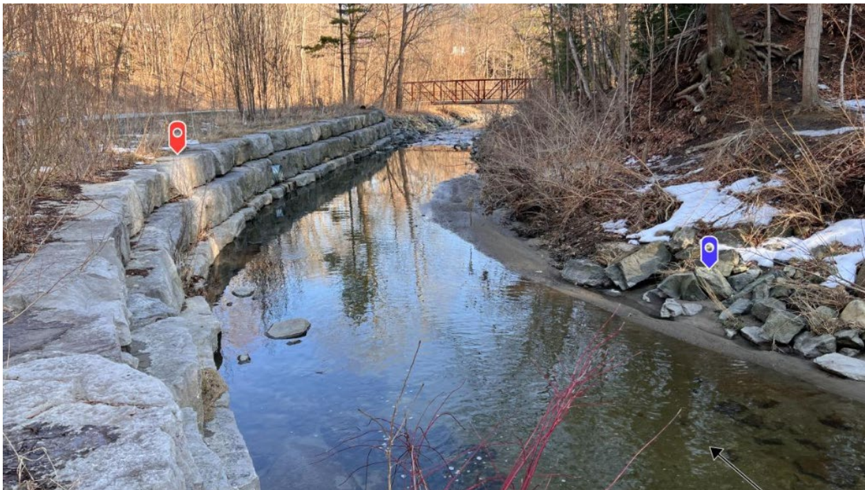
Figure 3. Armour stones (red marker) and riprap (blue marker) that have been placed along the river to mitigate erosion, at Stop #5 on the Wilket Creek Urban GeoWalk.
