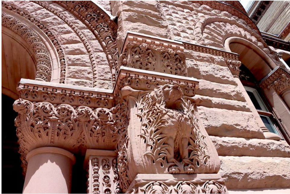
Figure 4. Whirlpool Sandstone at Old City Hall on the Downtown Toronto Urban GeoWalk.
