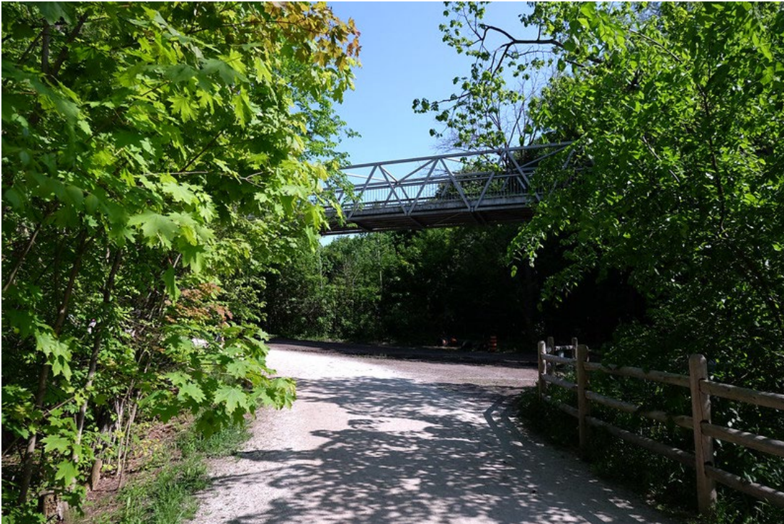
Figure 3: Heath Street Bridge (also called Cat's Eye Bridge) at Stop #2.
