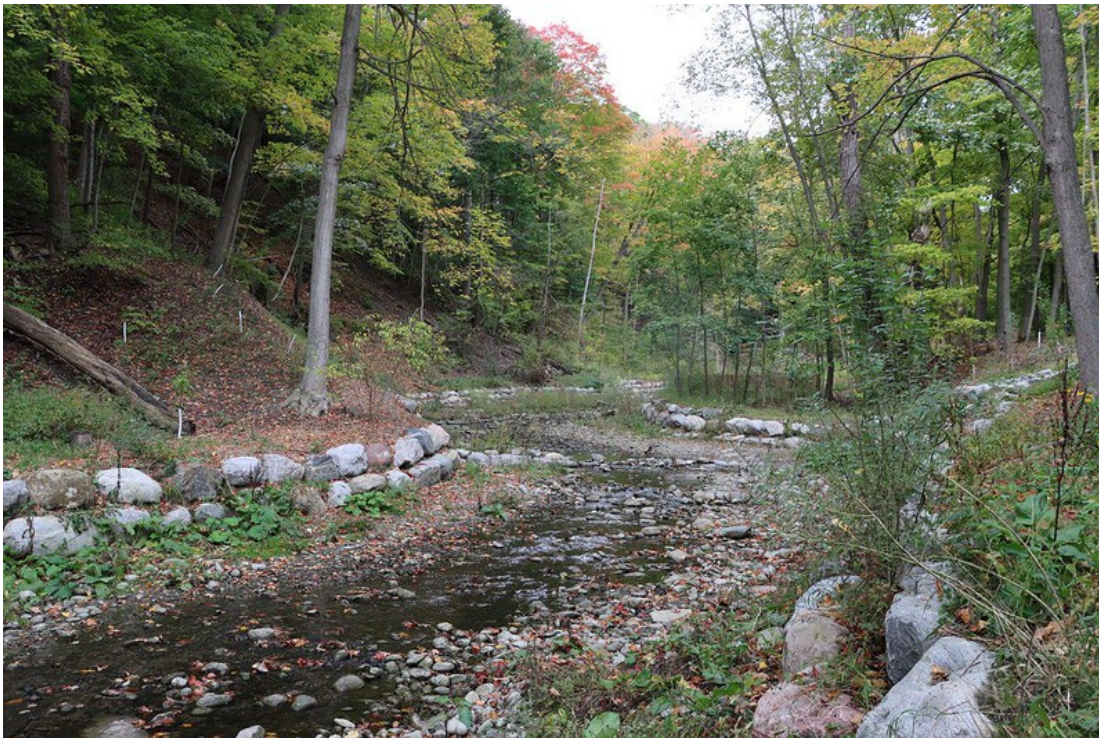
Figure 5: Boulders placed along Mud Creek to stabilize the banks at Stop #4.
