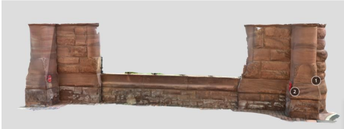
Figure 1: 3D LiDAR Model of The West Entrance Wall: Legislature Bldg.
