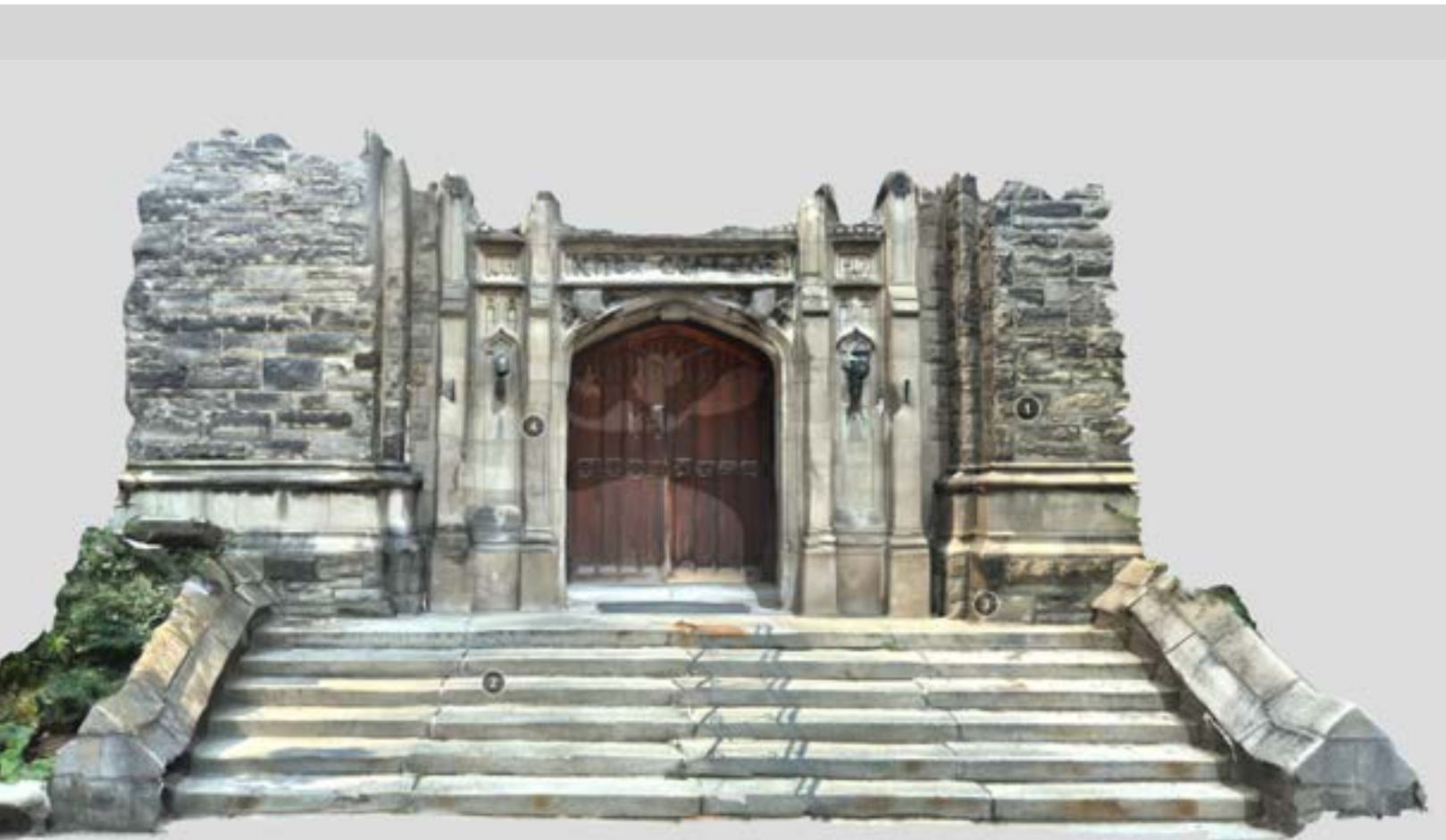
Photo: 3D interactive model of the east entrance of Knox College at the University of Toronto campus.
